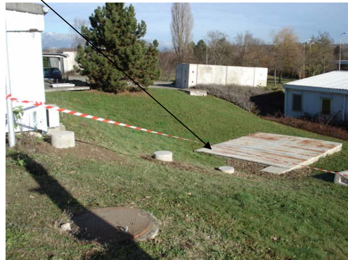
Concrete support posts for transfer line
