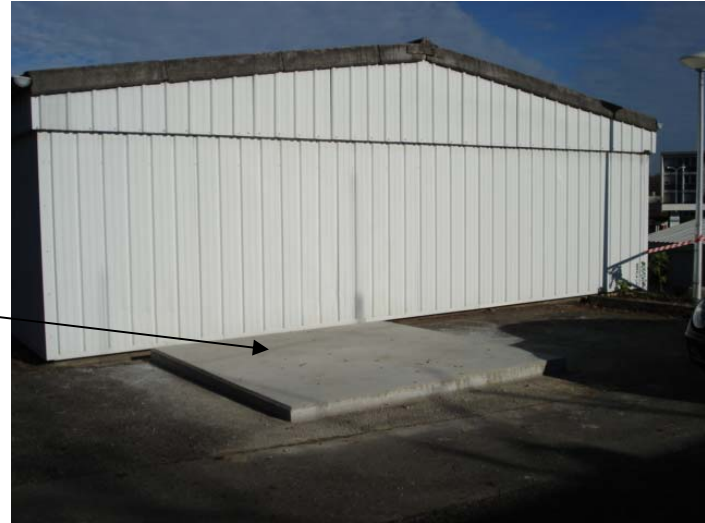
Concrete platform for dewar
