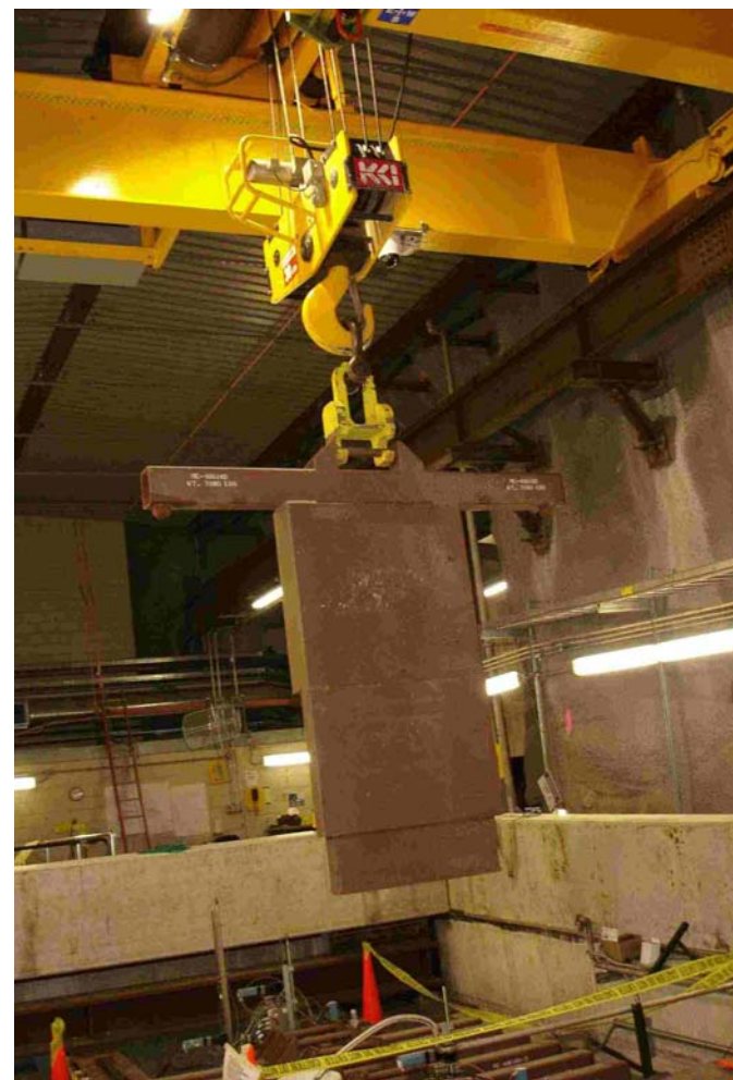
Steel shielding block being moved.
