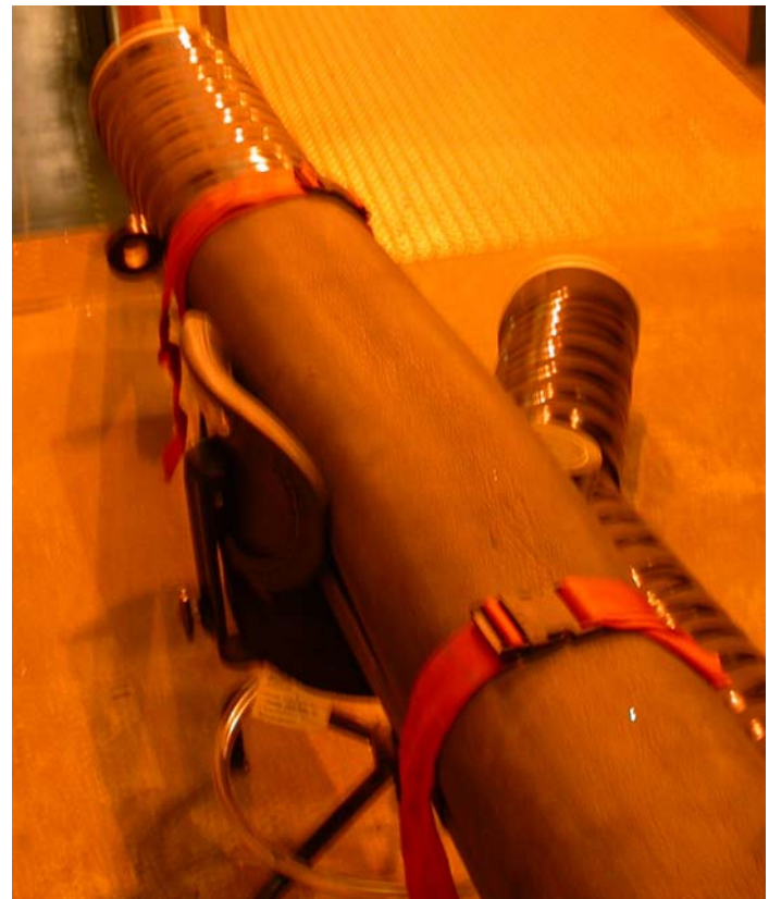
Insulating the top (roof) segment of the vent line
