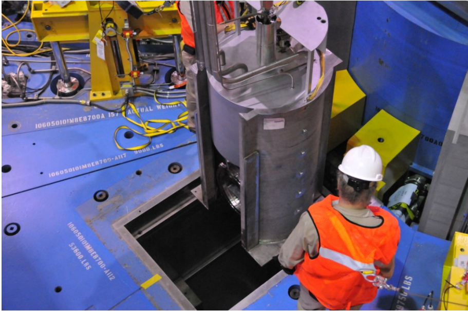
New PBW with guide can and counterweight being installed
