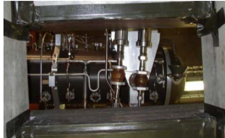
View of Horn 1 through shielding slot
