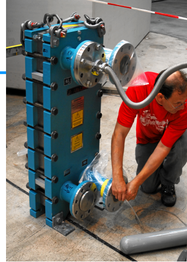
He leaktest of repaired Moderator HX
