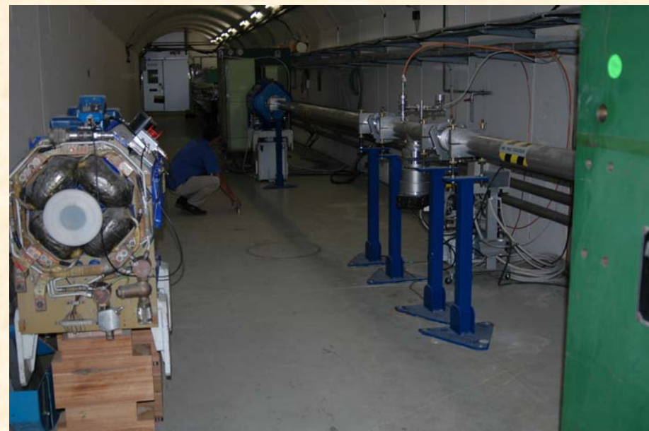
Tunnel Width 400cm (158")
