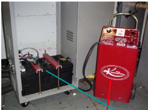
Battery/Charger 12V 1400A
