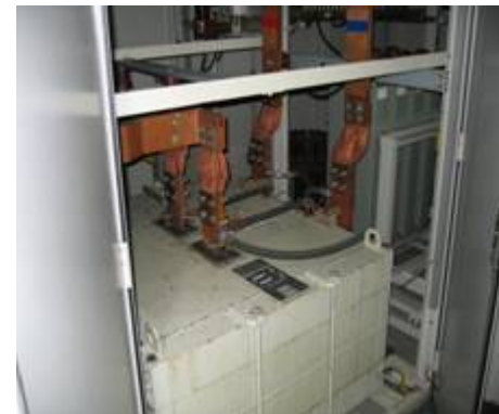
Passive filter capacitors
