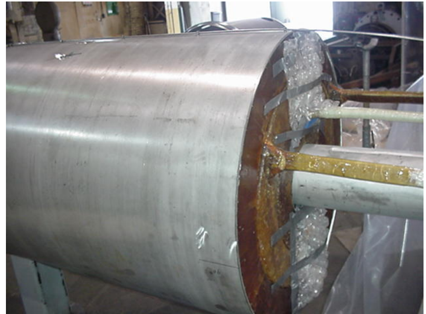
Coils inserted into pressure vessel September, 2005
