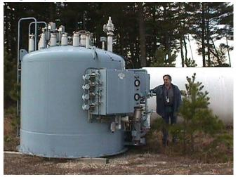
Fig. 4. The SSC-surplus heat exchanger for possible use in the proposed cryogenic system.
