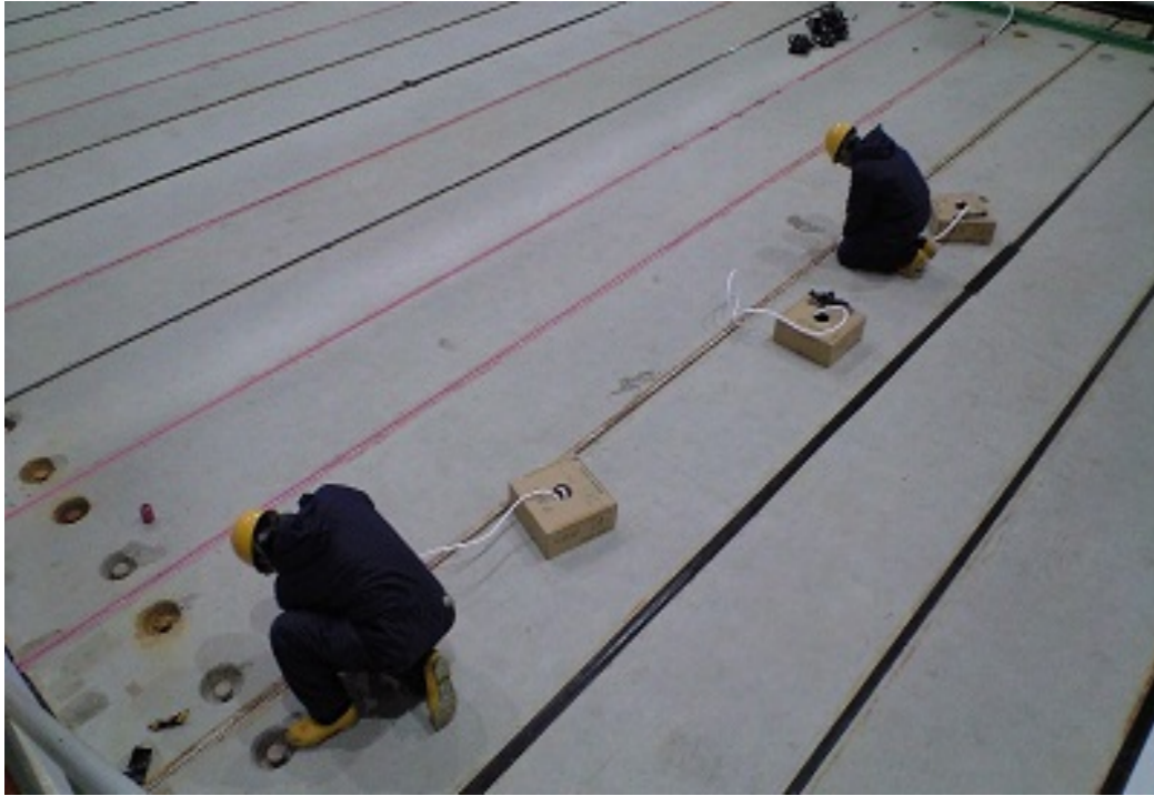
Caulking between concrete shields
